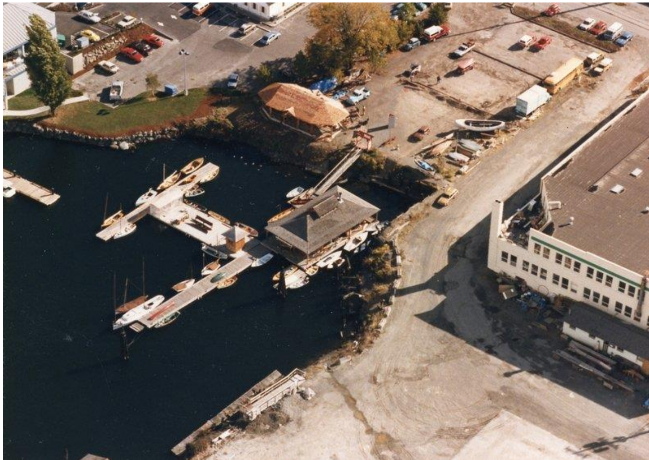
Aerial Image of Waterway 4, by Phil Webber, c. 1985, CWB Collection
