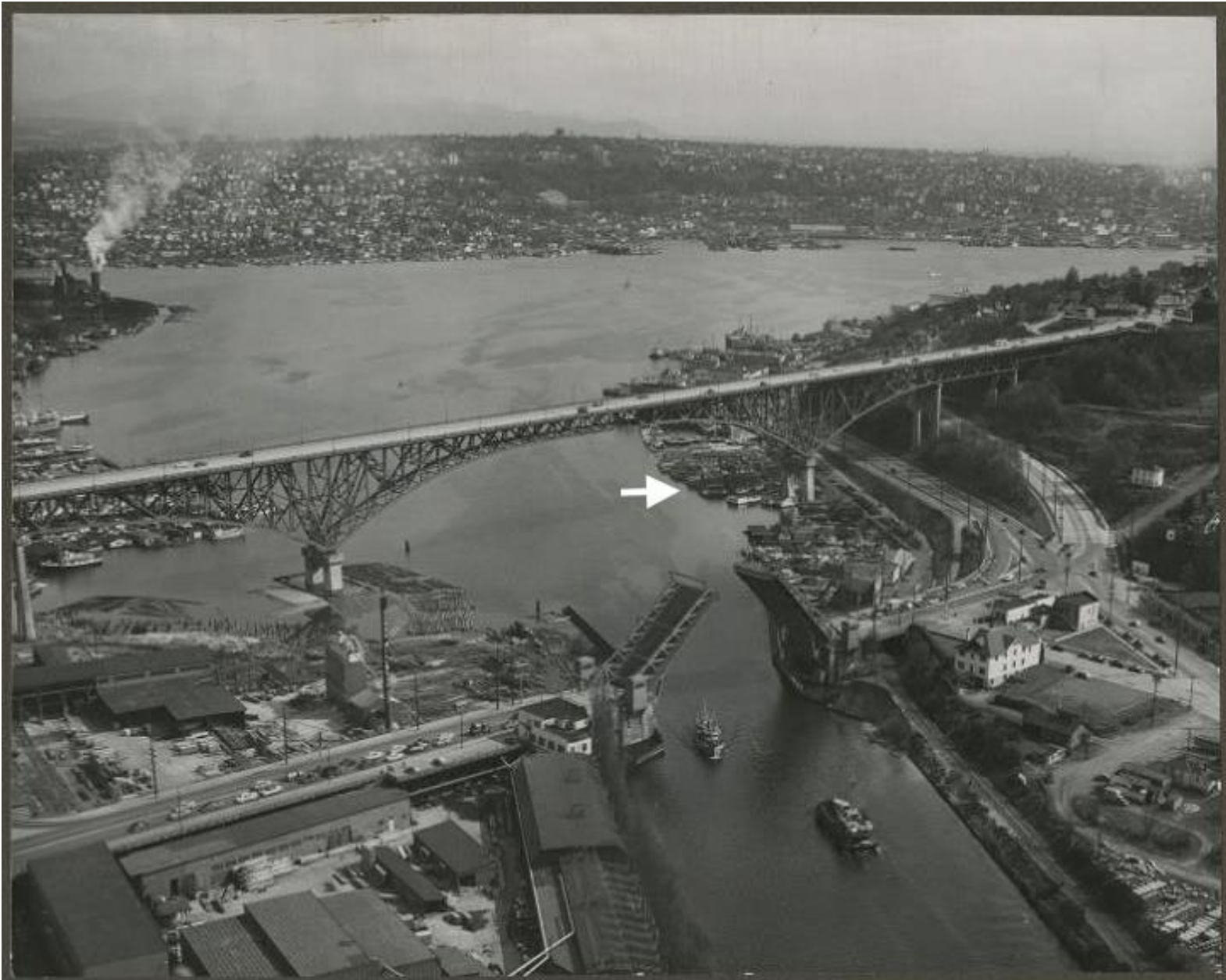
Aerial Photograph of George Washington Memorial Bridge (Aurora Avenue), 1950, Seattle Public Library
