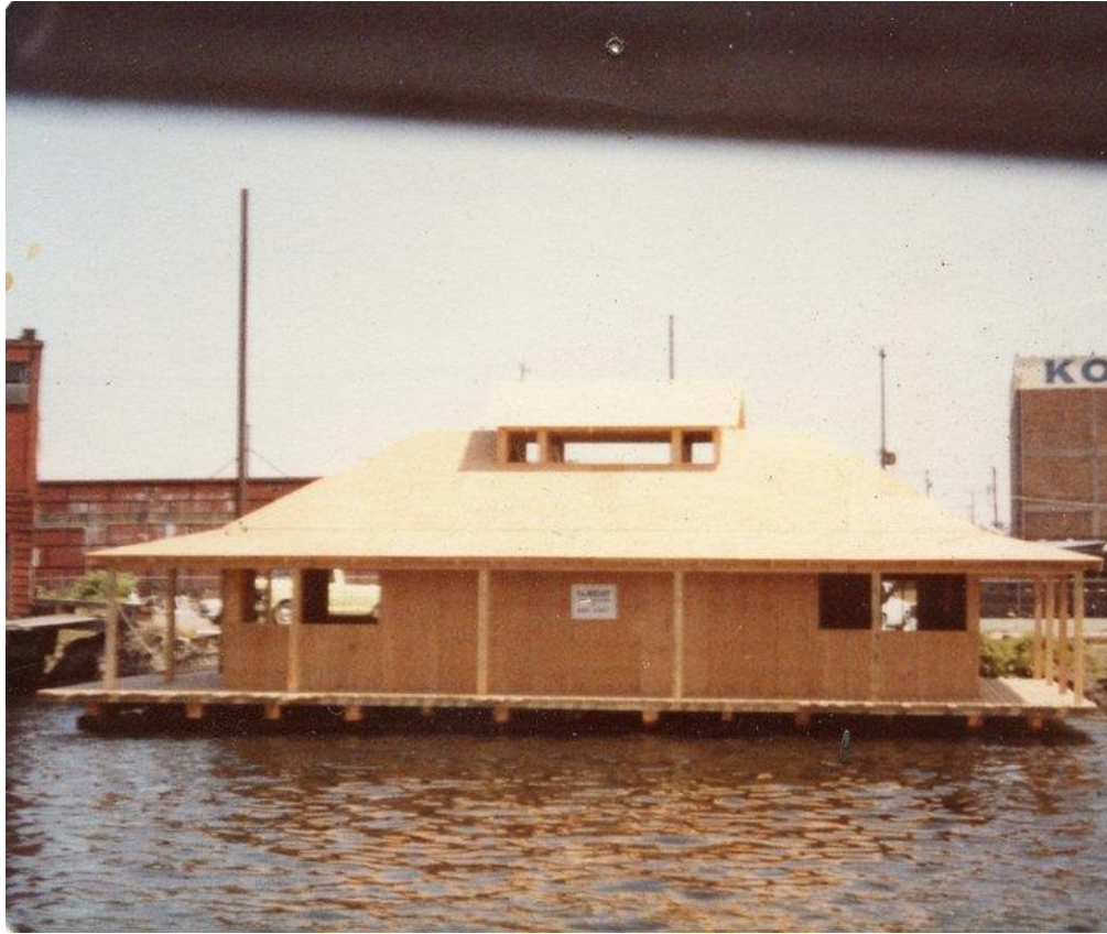
Boat shop under construction, 1982 or 1983, CWB Collection
