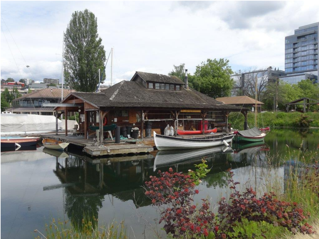
C13. View of north side of boat shop, showing gantry and sliding doors, view south, June 4, 2020
