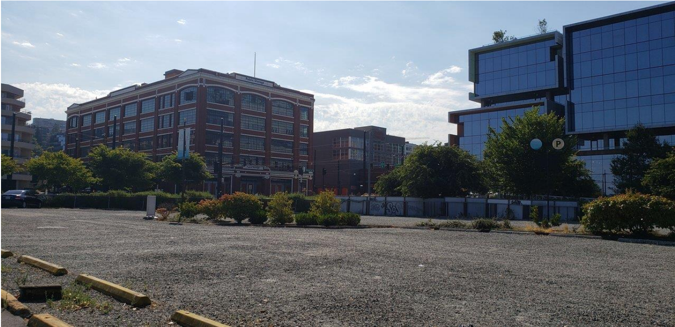
C3. View southeast of properties across Valley Street, including the 1913-14 Ford Motor Co. bldg. (left)
