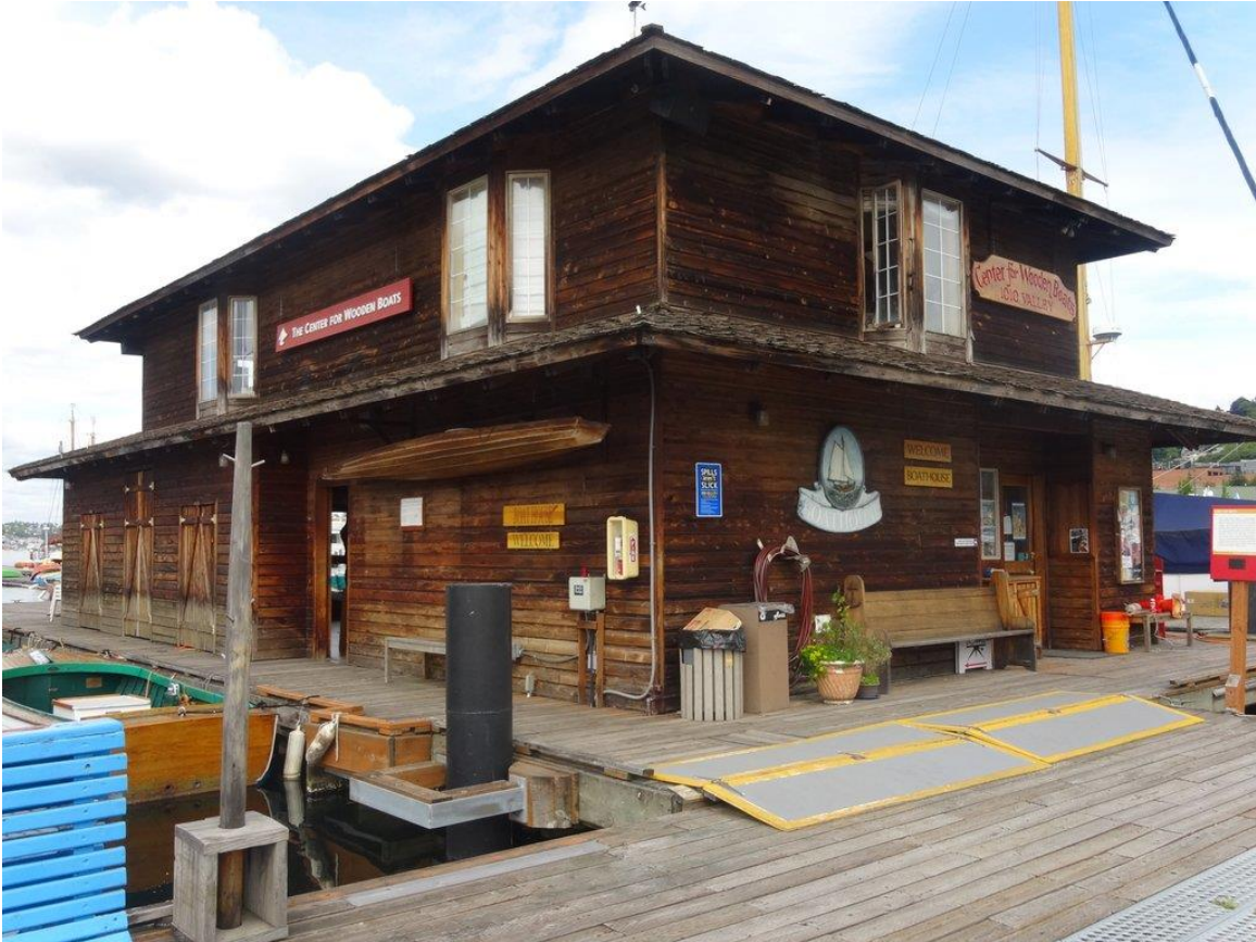
C19. Boathouse view of southwest corner; note the black steel piling in foreground, June 4, 2020
