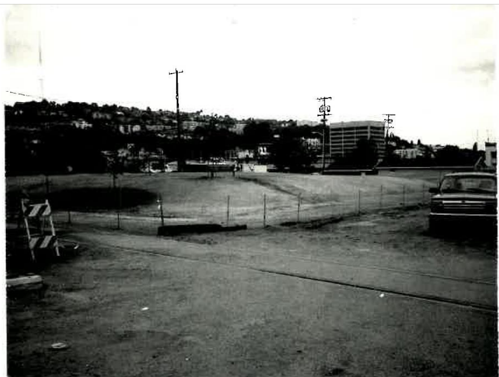
B25. Site of the former Belknap Glass building shortly after demolition, 1990. Source: King County Assessor.
