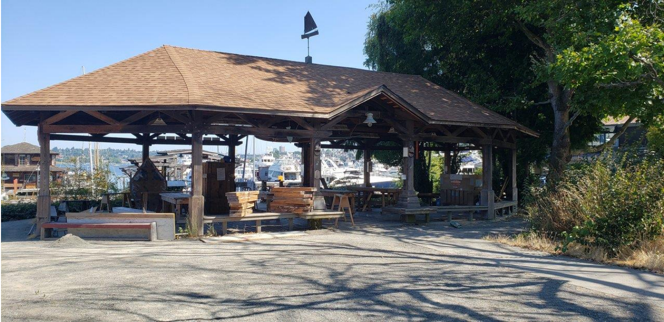
C24. View north showing the pavilion, August 16, 2020
